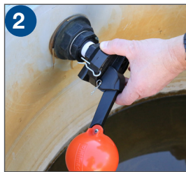
2 Screw in the float valve by hand, valve is suitable for final tightening with a wrench
