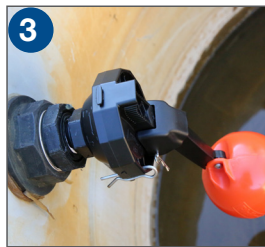
3 Ensure float valve is in the vertical position
