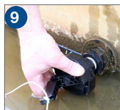
9 Screw float valve into position and thread string through plastic tube and attach to float
