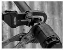
**3.** Using a pipe wrench or multigrips on the end caps only, further screw the air relief valve into the male thread until tight. Where necessary ensure the male thread is held stationary to avoid it from moving.
