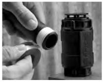
I. Apply PTFE tape or approved sealant to the male thread the air relief valve is to be screwed into. Sufficient tape needs to be applied to ensure a watertight seal.
