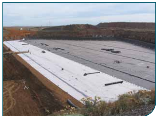
Geotextile Exposed
