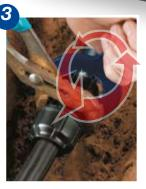
Tighten the nut by hand, and then with a wrench to the point where the nut is touching the flange on the body of the fitting. Do not tighten beyond this point.
