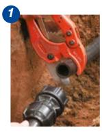
Cut the pipe square, there is no need to chamfer or lubricate the pipe.
