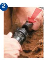
Ensure 2 threads are showing and simply slide the pipe in until the first point of resistance is felt.
