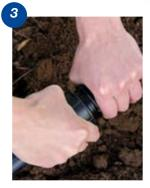
Tighten the nut by hand (up to 25mm) or with a wrench.
