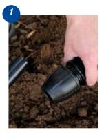
Cut the pipe squar. There is no need to chamfer or lubricate the pipe. Ensure 3 threads are showing.
