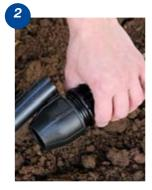
Slide the pipe into the fitting until the first point of contact is felt. There is no need to force the pipe in.
