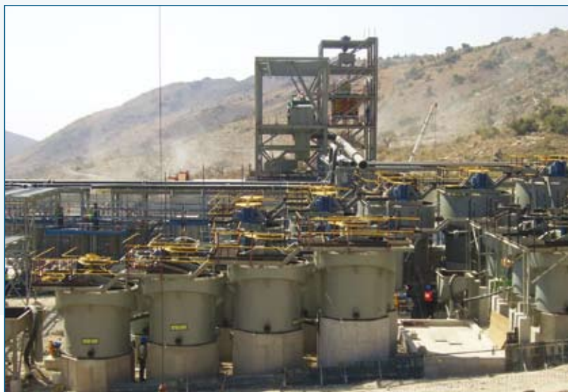
Flotation section of Processing Plant.
