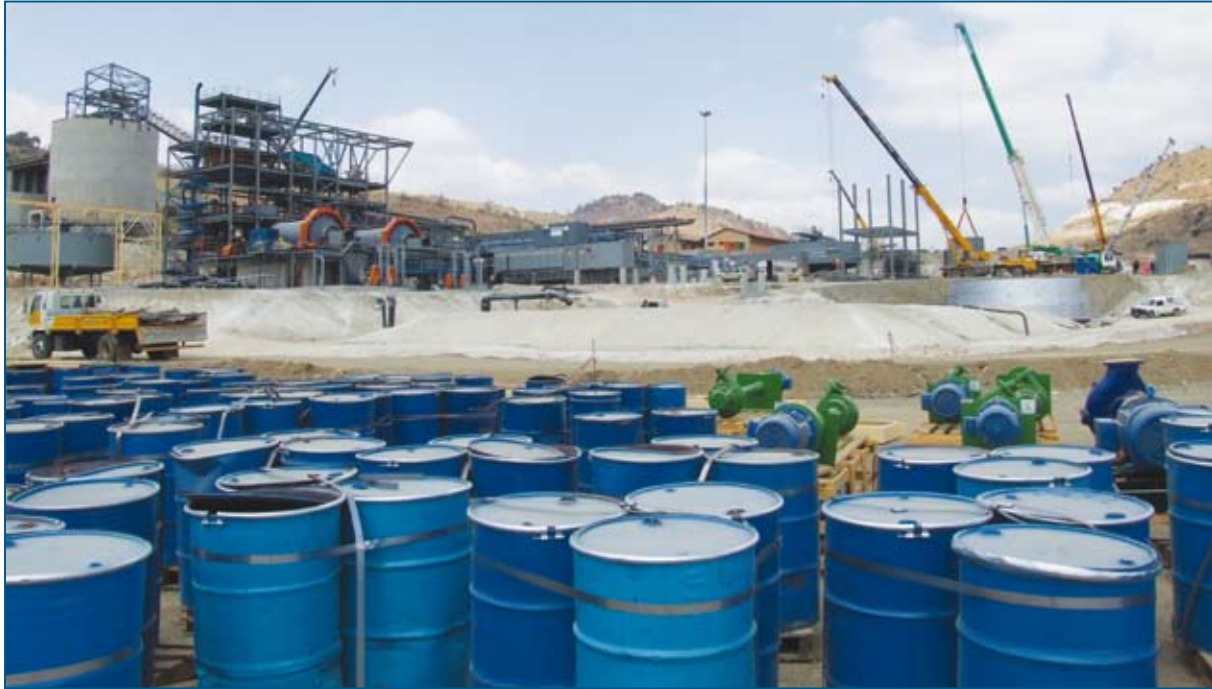
Smokey Hills Processing Plant nearing completion.
