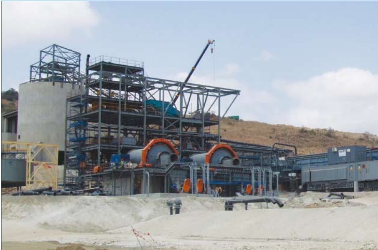
Milling section of Processing Plant at Smokey.
