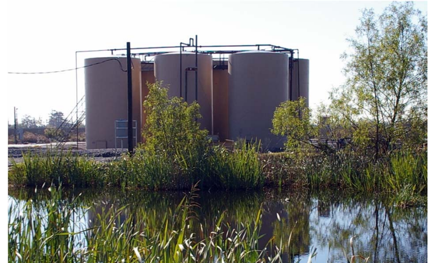
East Chalkley Tank Battery
