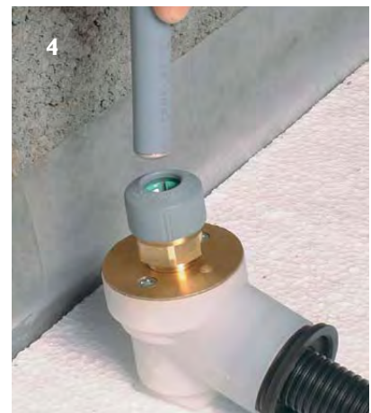
Pipe push-fitted into Hep 2 O ® adaptor.
