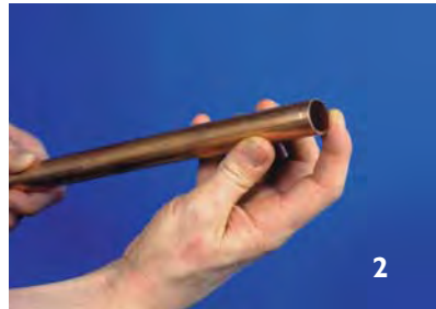
Inspect ends to ensure they are free from burrs or swarf
