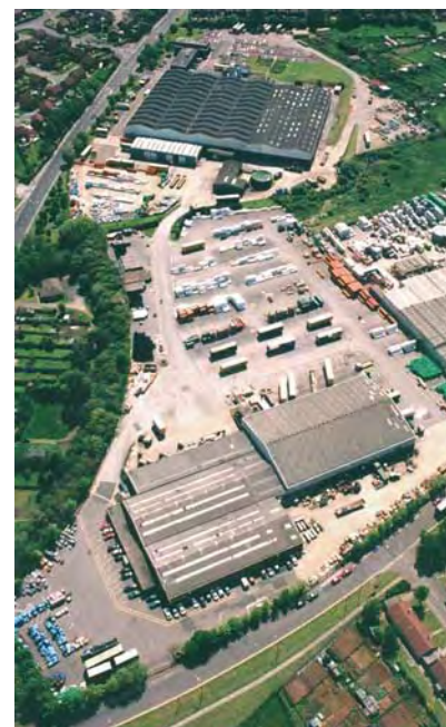
Hepworth's Doncaster manufacturing plant
