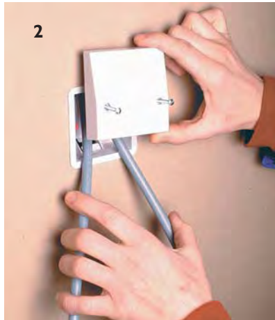
The HX111 Cover Plate is screwed to the back-plate.
