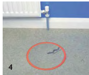
The chipboard cut-out fits snugly into the Routabout Spacer Ring, leaving a neat access.
