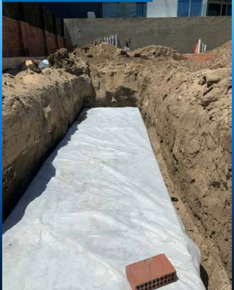
Tank Wrapped, Ready For Backfill
