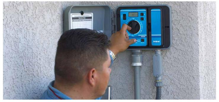
We've upgraded these popular, long-standing controllers with a host of new features. The Irritrol<sup>®</sup> Rain Dial-R now offers exceptional scheduling for speed of programming and maintenance. Additional features include rain sensor compatibility and more pump control for water well and booster pump applications. And best of all, the new Rain Dial-R programs just like the original-use only the features you need!
