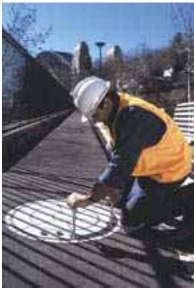
Decorative edge can be attached to the cover and frame for aesthetic areas. This adds 12mm or 40mm to overall height to accommodate tiles or pavers
